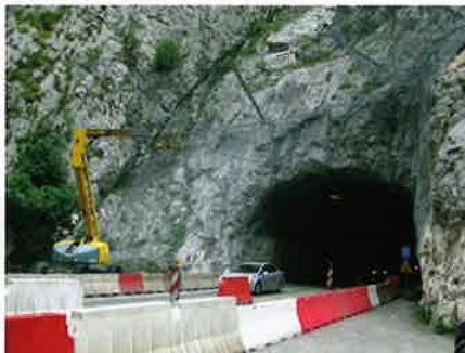
Fig. 2. Securing of a portal in rock in Macedonia (photo: Geobrugg)
